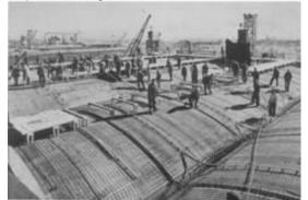
8) Ferrocement or Ferrocrete works where WWR is the only solution for forming the reinforcing matrix along with chicken mesh to develop thin and efficient precast elements such as water tanks, fins, shelves etc.
